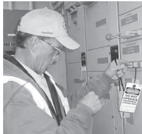
Lead mechanic Harry Stites performing LOTO.
